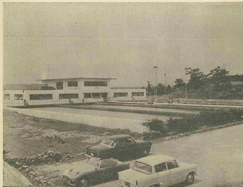
TYBASE WATER TREATMENT PLANT
