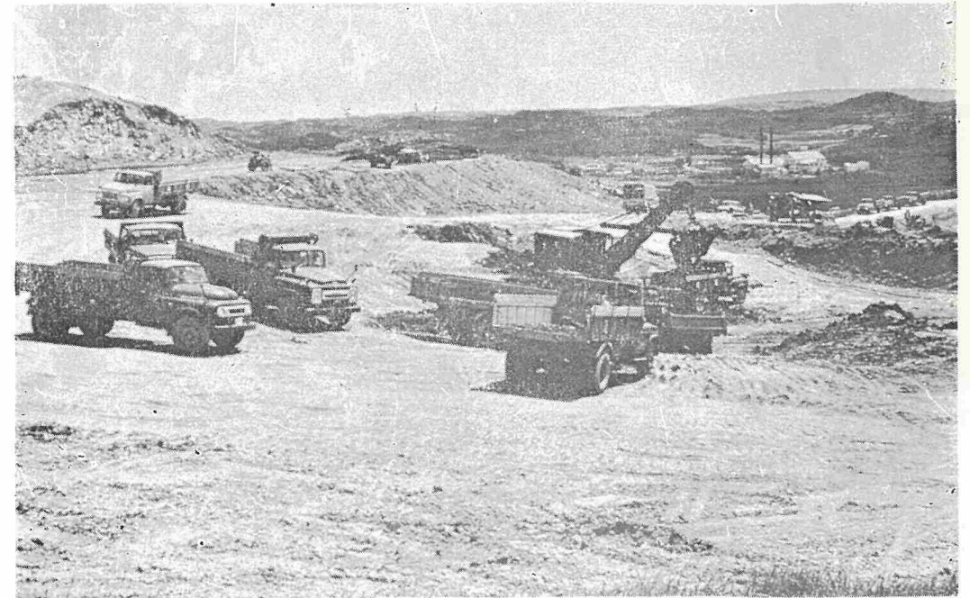
Grading site of the Naha water Storage facility.
