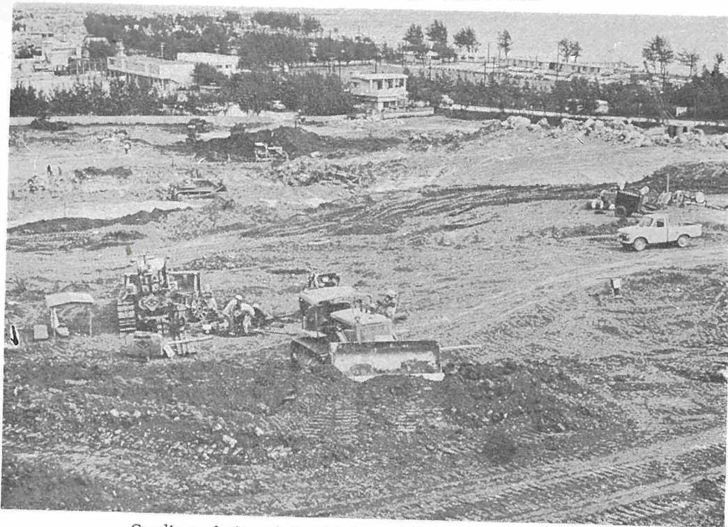
Grading of site of the Ishikawa Water Treatment Plant.
