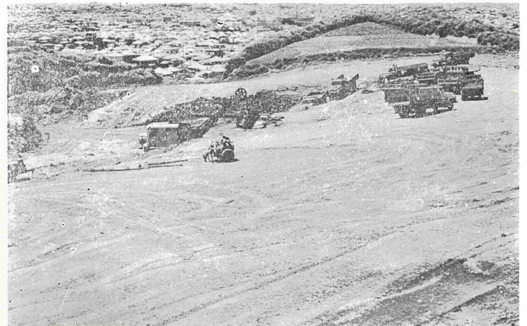
Construction site of Naha Water tank with Naha harbor in the background.
