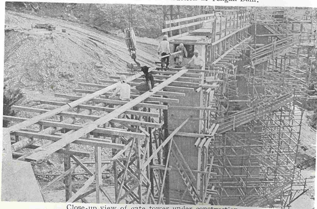
Close-up view of gate tower under construction.
