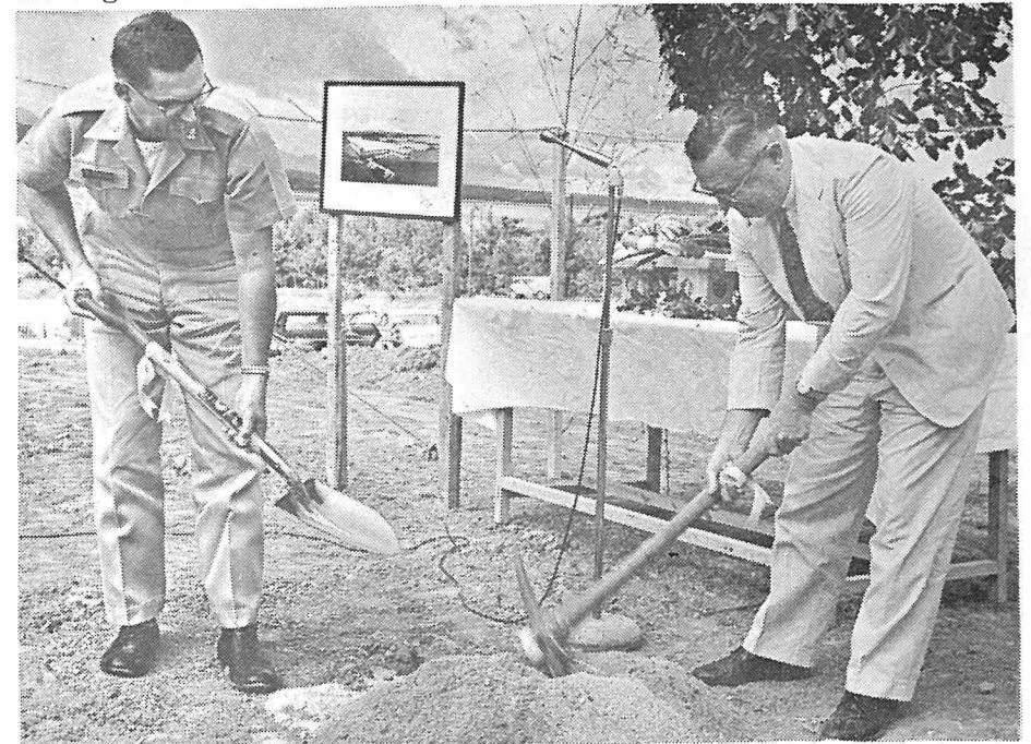
Lt. Col. William H. Beauchamp (right), the Alternate Board Chairman for RDWC and Maj. Richard B. Boughton, (let), U.S. Army Engineer District, Okinawa actively engaged in th ground-breaking ceremony for the new water treatment plant at Ishikawa
