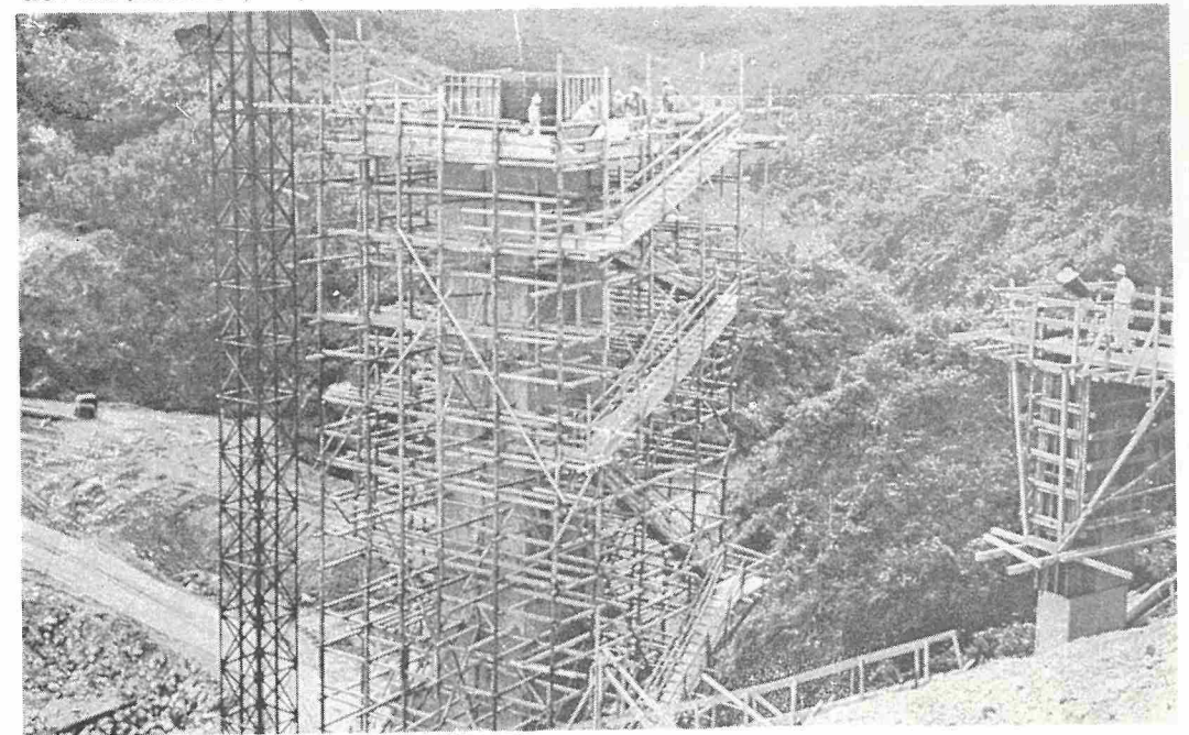
View of the gate tower under construction.
