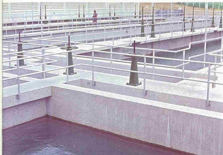
Flocculation basin, sedimentation basin and filter
