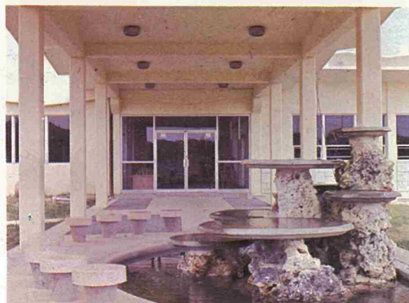
Front entrance of the plant
