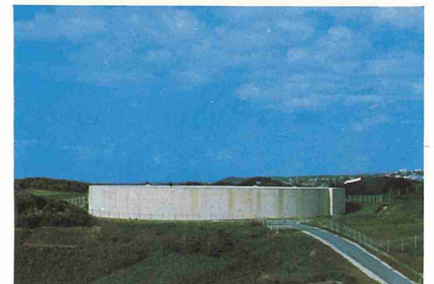
General view of 10 MG Naha Storage Tank
