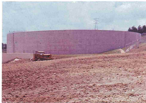
10 MG raw water storage tank for the plant
