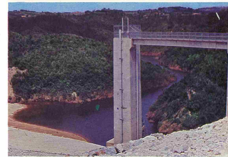
Control tower of Tengan Dam
