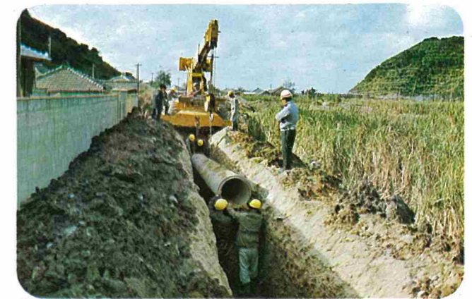
Pipe installation at Genka
