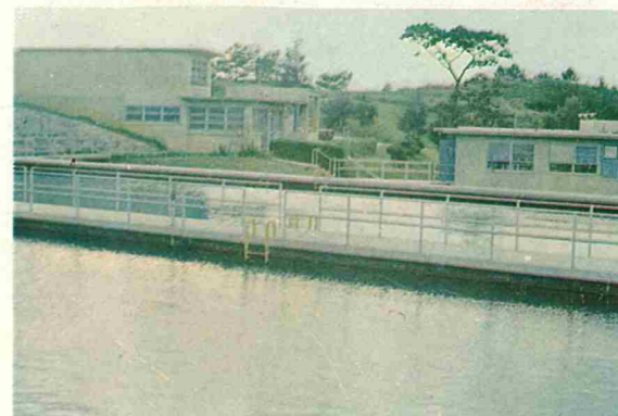
Tengan Treatment Plant
