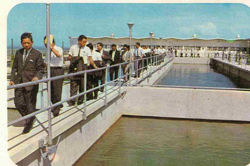
The visitors touring the Ishikawa Water Treatment Plant.
