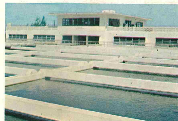
Tybase Treatment Plant
