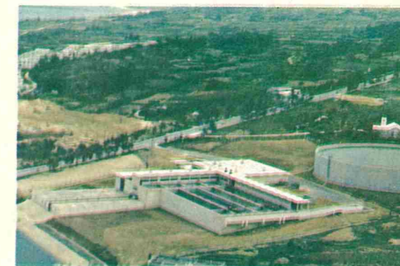
Ishikawa Treatment Plant
