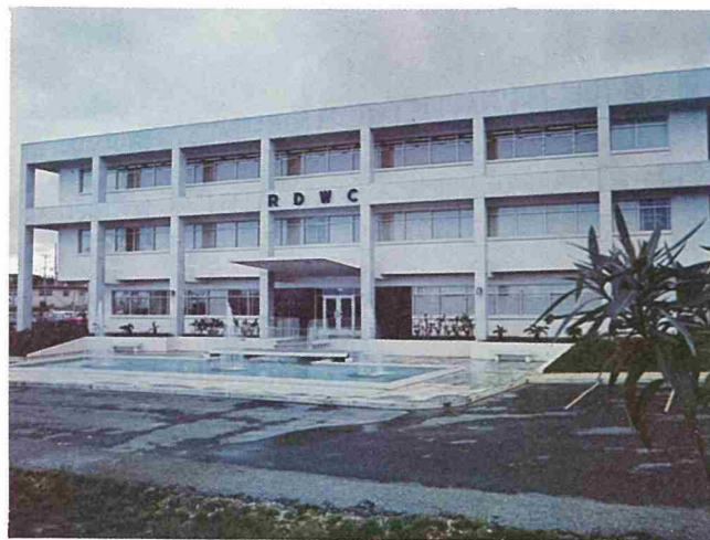
RDWC's NEW HEADQUARTERS
