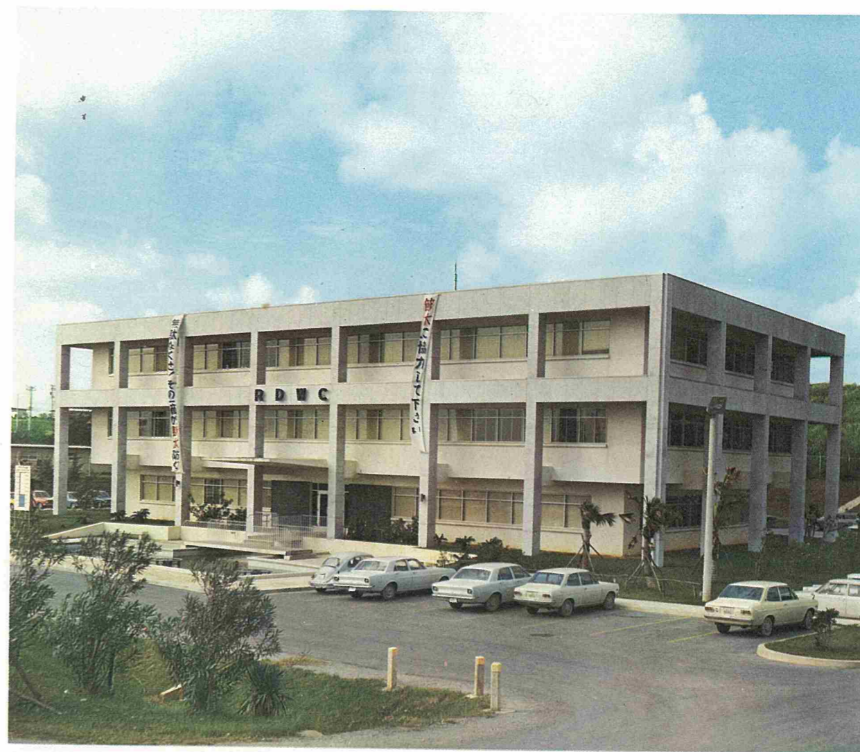
The office building with a total floor space of 23,135 square feet was completed in July 1970.
