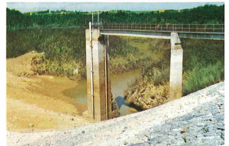
Tengan Dam and Reservoir
