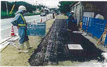
LU型側溝(取壊し状況)
