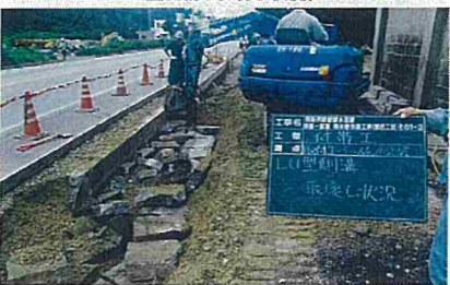
LU型側溝(取壊し状況)
